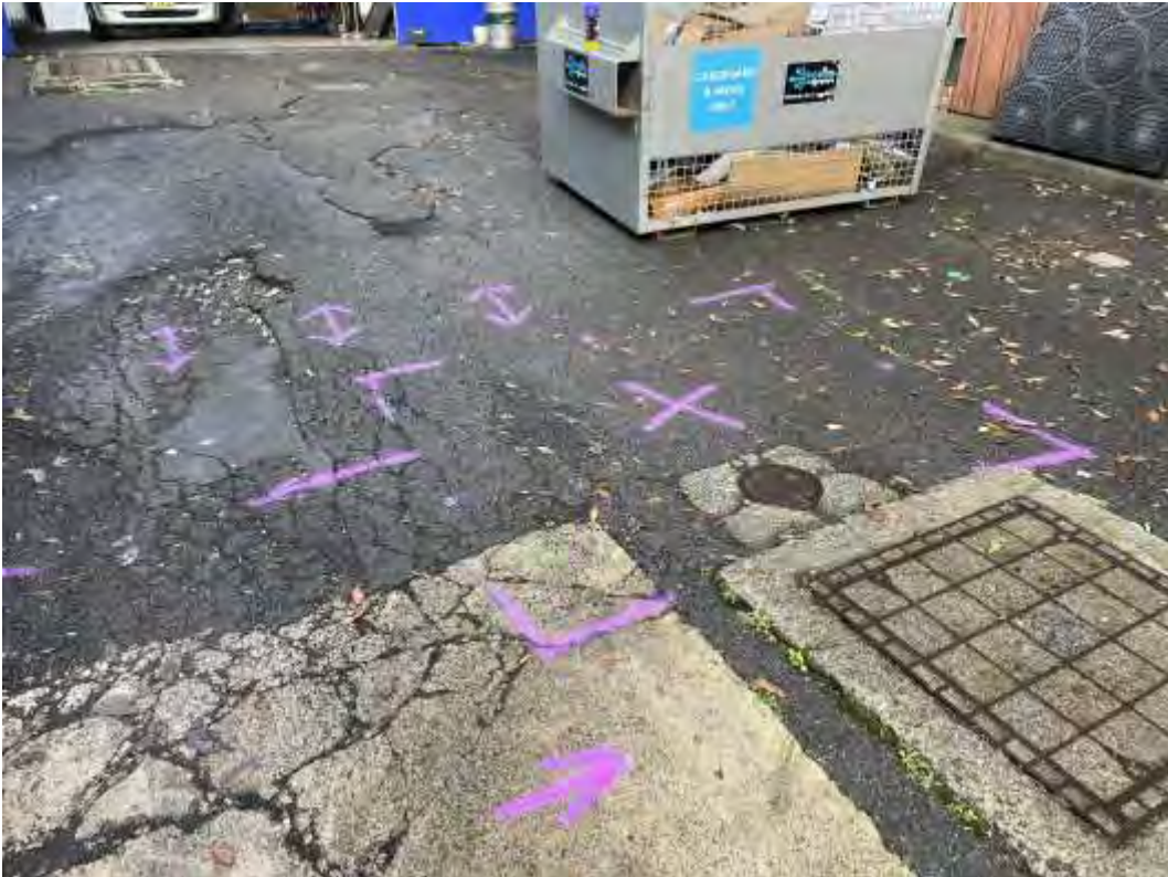
Photograph 5: Image of the approximate location of the UST (dated 5 June 2024).
