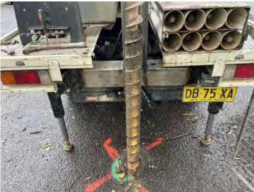
Photograph 10: Image of borehole BH11 (dated 5 June 2024).
