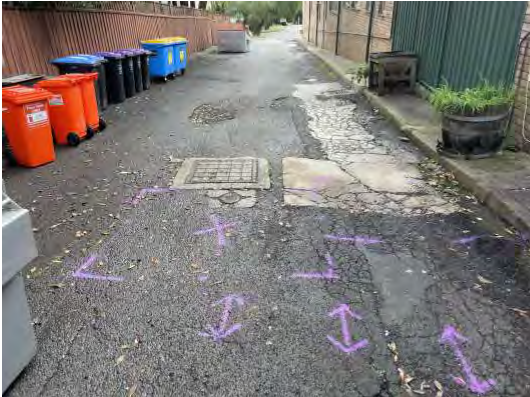
Photograph 7: Image of the approximate location of the UST and service locating showing potential underground piping, looking north (dated 5 June 2024).
