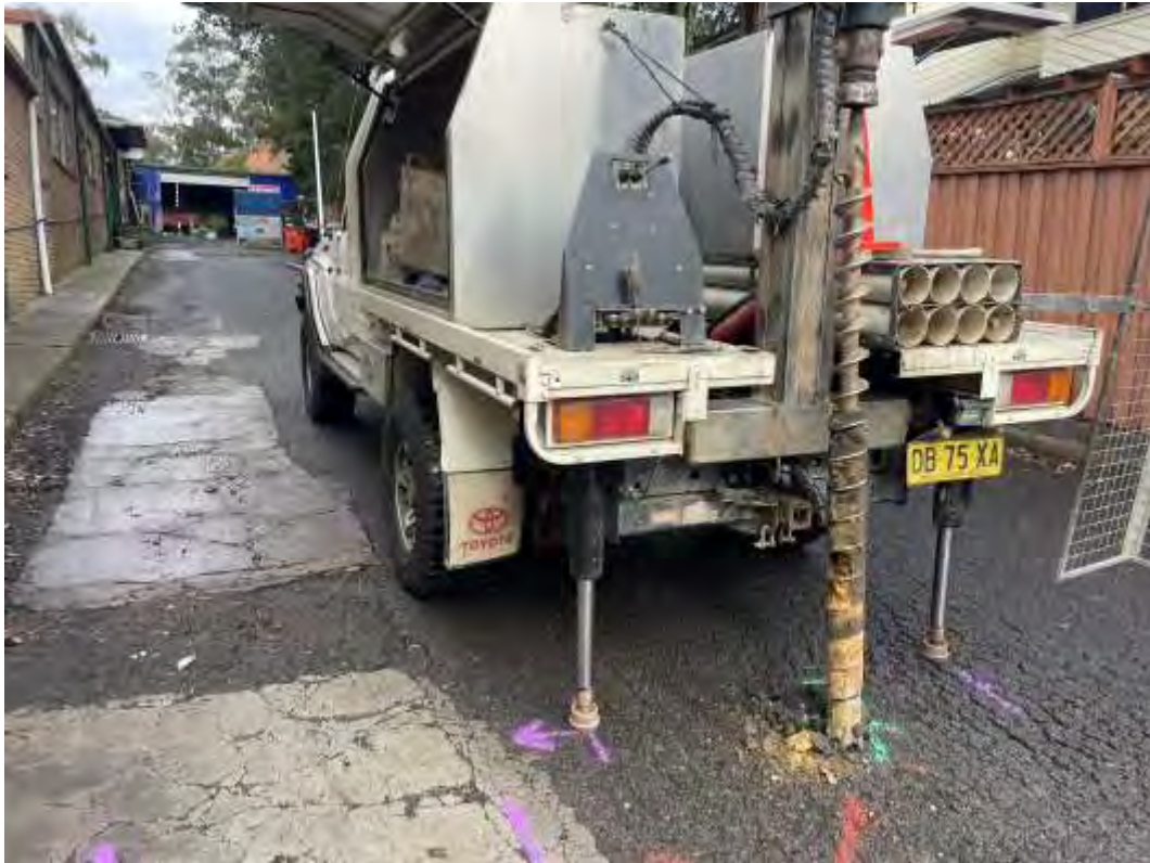
Photograph 11: Image of borehole BH16 (dated 5 June 2024).
