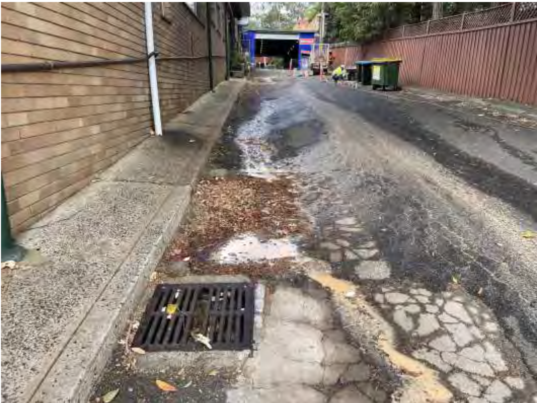
Photograph 4: Image of the western driveway, looking south (dated 17 October 2023).
